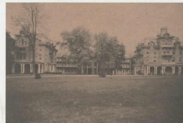
A turn-of-the-century photograph shows Norland Hall at left, Edgar Hall at right, and Main Hall between the two.
